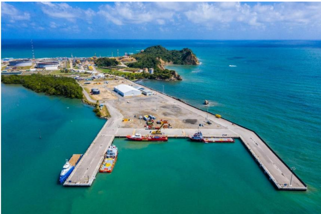
Figure 1: Aerial View of Port of Galeota
